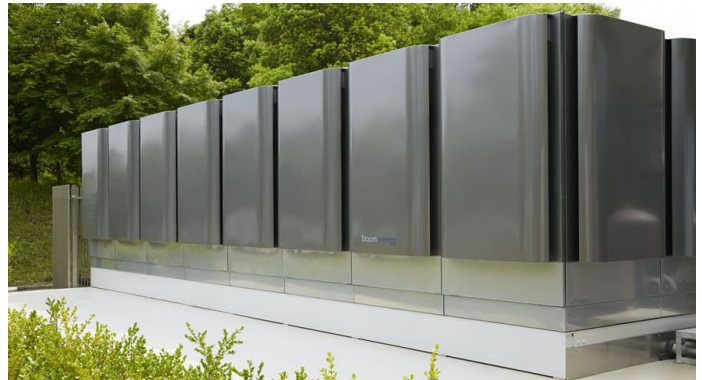
Fuel cells generate electricity without combustion through a chemical process.
